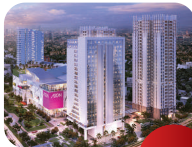
Apartment Southgate Jakarta
